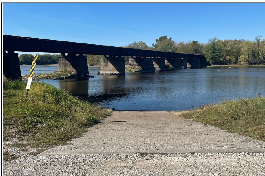
Looking west-southwest at Moscow Railroad Bridge from Langes Ferry Crossing, 2023
