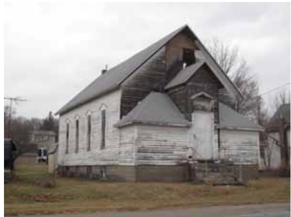
M.E. Church - 3885 Hwy 22 - Montpelier - MP-43
