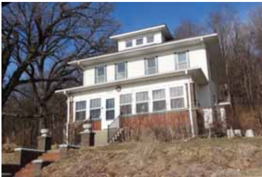
House - 2236 Burlington Road – FR-06
