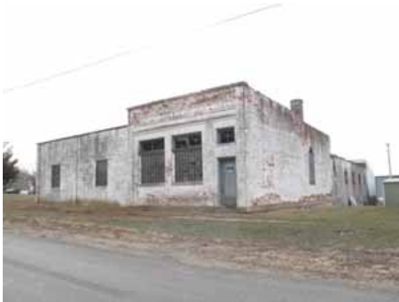
Building - 213 Commerce - Stockton - FL-36
