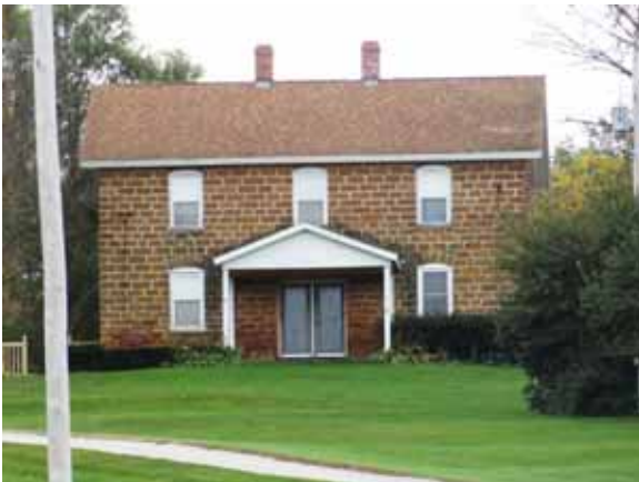
House - 3482 180th St - MP-12
