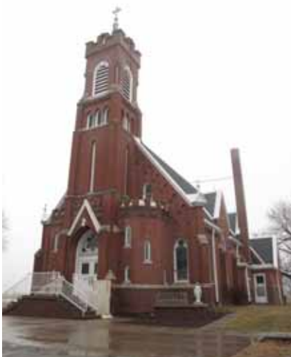
St Mary's Catholic Church - 414 Grand Ave - Nichols - PI-10
