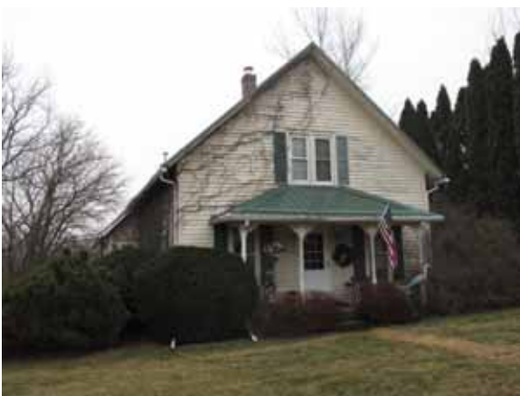
House - 2493 Fry Ave - Cranston - CE-11
