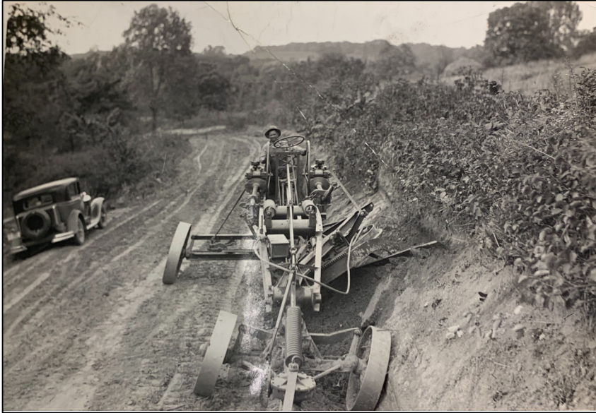
Figure 45. Widening a narrow uphill grade in Muscatine County, c.1940. Sources: Muscatine County Highway Department, Muscatine, Iowa
