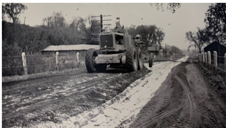
Figure 44. Heavy equipment spreading calcium chloride to help prevent freeze damage, c.1940. Source: Muscatine County Highway Department, Muscatine, Iowa
