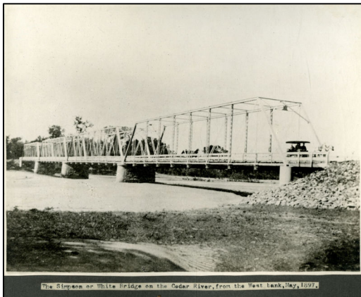
Figure 56. Left – Looking east from the west bank at the Simpson Bridge, built 1895, a Pratt through truss bridge, carried the Simpson Road, part of the Muscatine-Nichols Road, over the Cedar River. Right – The Iowa Highway 22 Bridge over the Cedar River. This Camelback through truss bridge replaced the Simpson Bridge in 1941. It was replaced again in 1987. Sources: Left - Musser Public Library. Part of the E. L. Graham Collection; Right – Muscatine Journal , December 30, 1940
