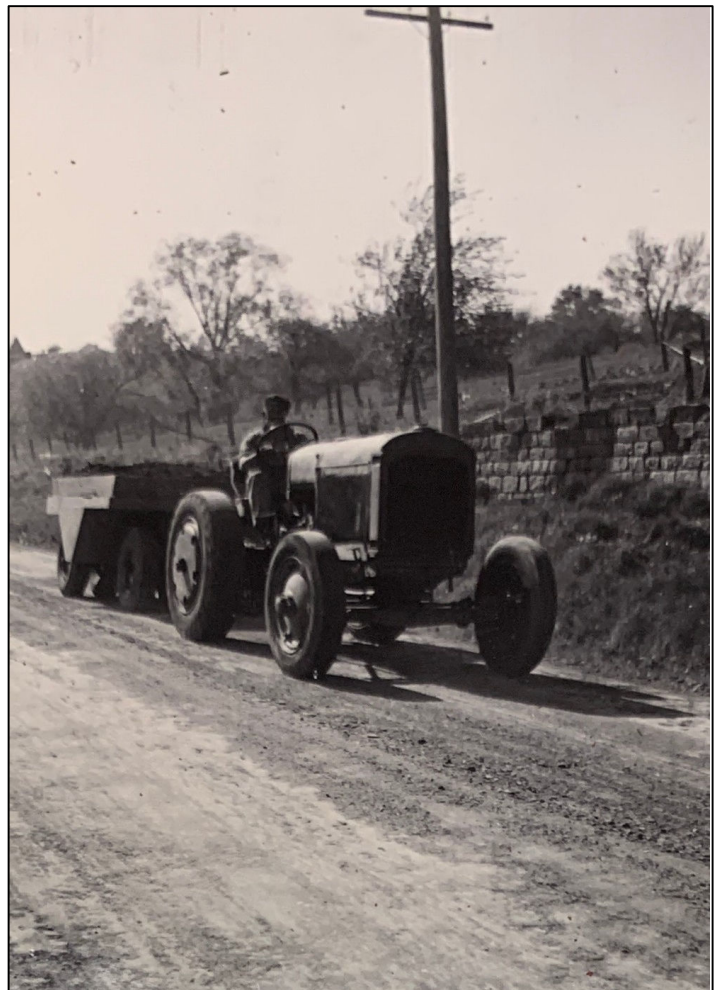
Figure 46. Compacting road surface with the pneumatic tire roller, c.1940. Source: Muscatine County Highway Department, Muscatine, Iowa
