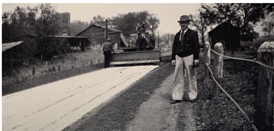
Figure 43. Spreading calcium chloride to help prevent freeze damage, c.1940. Source: Muscatine County Highway Department, Muscatine, Iowa
