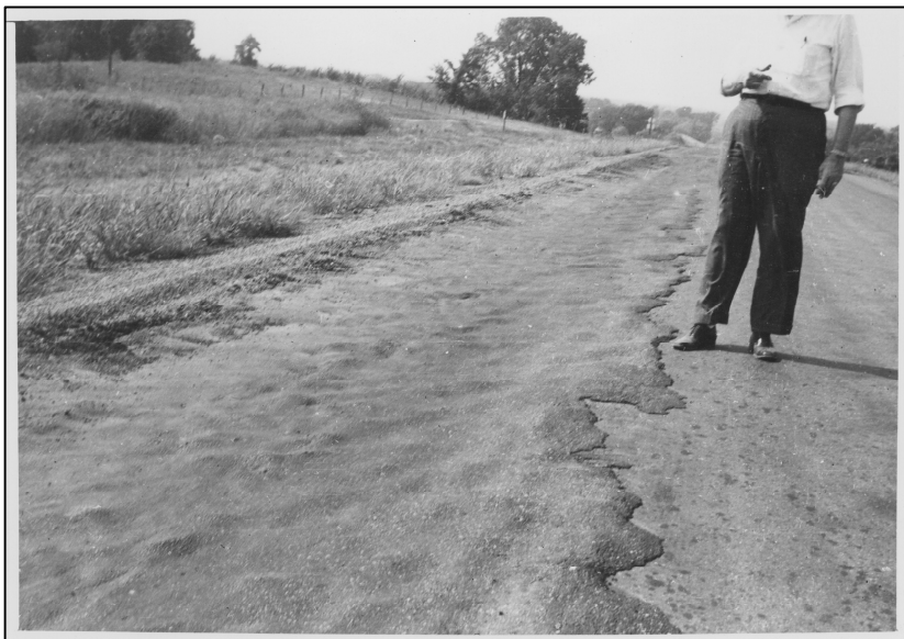
Figure 47. Examining an experimental soil cement stabilized base on State Highway 22 in 1947. Source: IHC Photographs Collection, Iowa DOT Historic Archives
