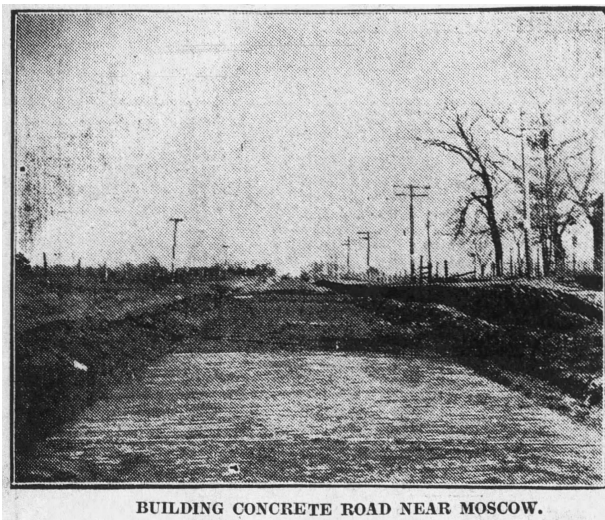
Figure 28. The concrete road segment (about four-tenths of a mile long) near Moscow along the River-To-River Road, was the first concrete-paved road in the county, and it is extant (TR-MS-07). Source: Muscatine Journal , December 12, 1914
