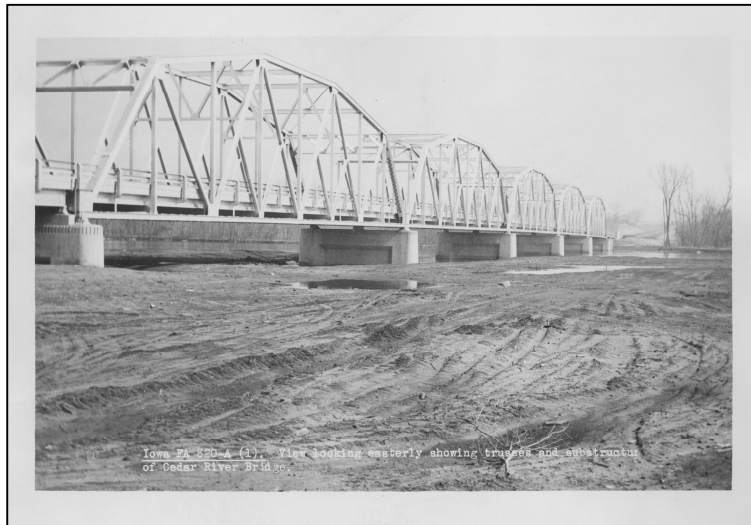
Figure 57. Looking upstream at State Highway 22 Bridge over the Cedar River was a five-span Camelback through truss bridge completed in 1941. Source: IHC Photographs Collection, Iowa DOT Historic Archives
