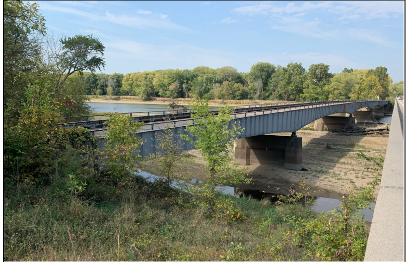
Figure 55. McKeown Bridge, 2012, a haunched steel girder bridge over the Cedar River on the former alignment of 231st Street. It was completed in 1951 to replace the 1879 McKeown Bridge, the first permanent bridge over the Cedar River. It is now a pedestrian-only bridge. Photo by Lynn Pruitt, Muscatine County HPC
