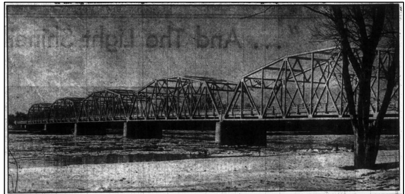
Figure 56. Left – Looking east from the west bank at the Simpson Bridge, built 1895, a Pratt through truss bridge, carried the Simpson Road, part of the Muscatine-Nichols Road, over the Cedar River. Right – The Iowa Highway 22 Bridge over the Cedar River. This Camelback through truss bridge replaced the Simpson Bridge in 1941. It was replaced again in 1987. Sources: Left - Musser Public Library. Part of the E. L. Graham Collection; Right – Muscatine Journal , December 30, 1940
