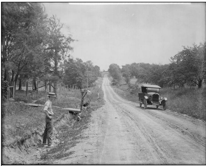
Figure 40. Typical improved graveled-surface road, 1925. Source: Musser Public Library, Muscatine, Iowa
