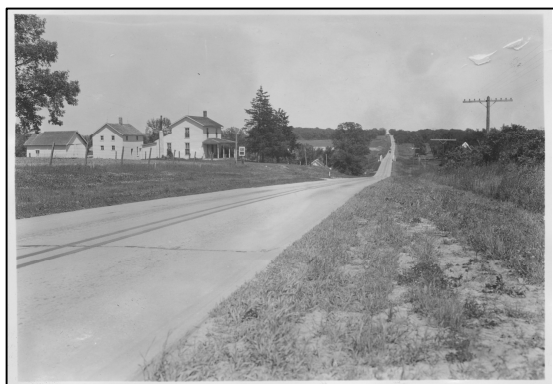
Figure 39. Early paved section of US Highway 32 west of West Liberty, probably 1928 when paving from the Johnson County line east to West Liberty was completed. Source: IHC Photographs Collection, Iowa DOT Historic Archives
