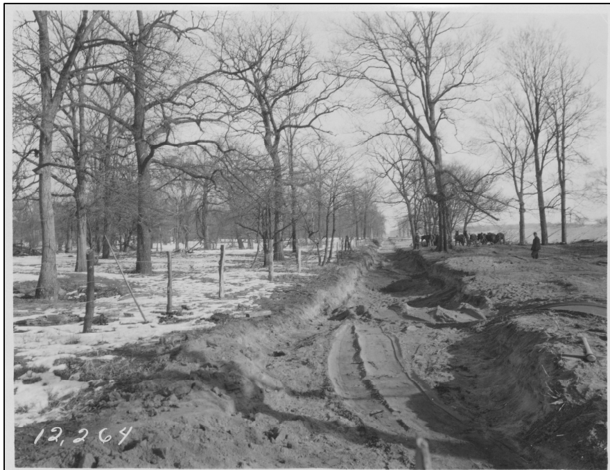
Figure 32. Typical condition of an unimproved road in 1928. Source: IHC Photographs Collection, Iowa DOT Historic Archives
