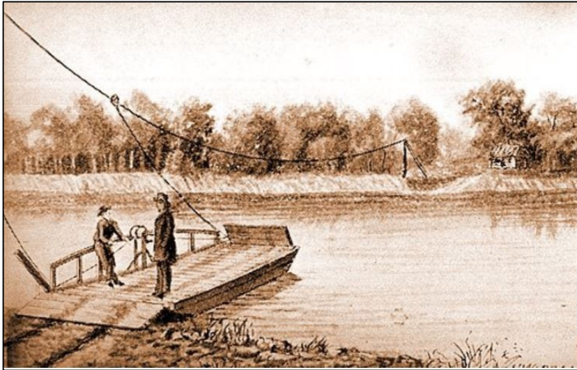
Figure 10. An example of a rope ferry with “comfort station” on opposite shore. This was the basic operation of Lange’s Ferry after he took over for William Slater in 1852. Source: Revolutionary War Journal website
