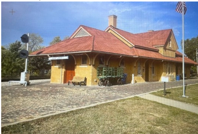
TR-WA-05 West Liberty Rock Island-BCR&N Railroad Depot 41.571395, -91.267959
